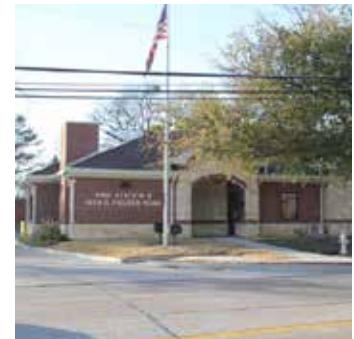
Station 6 Fielder Rd
