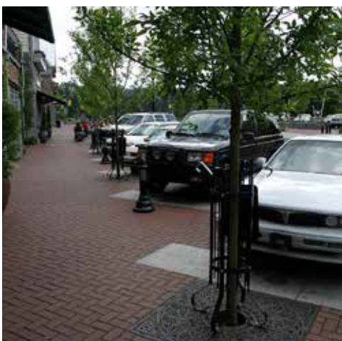
Parking constructed with pervious material
