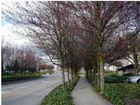
Sidewalk meander around trees
