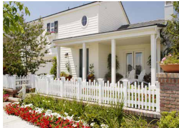
Territorial reinforcement – physical elements such as fences, pavement treatment, signs, and landscaping define clear boundaries between private and public spaces
