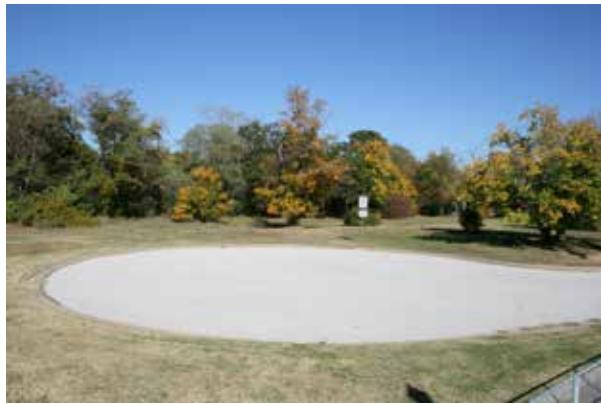
Street pavement remaining in Julia Burgen Park
