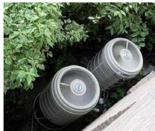
Outdoor components of a residential heat pump
