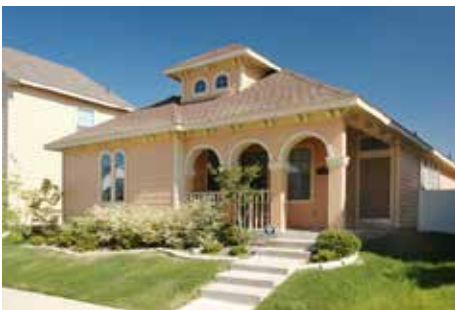
Light colored building materials
